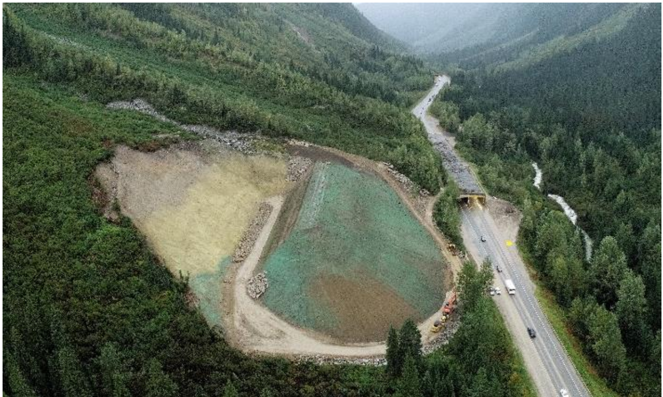
Figure 7. Constructed Mounds catchment and stopping berm, which measures 18.5 m high by 150 m long. The Single Bench snow shed can be seen immediately downslope and east (photo right) of the toe of the berm.
