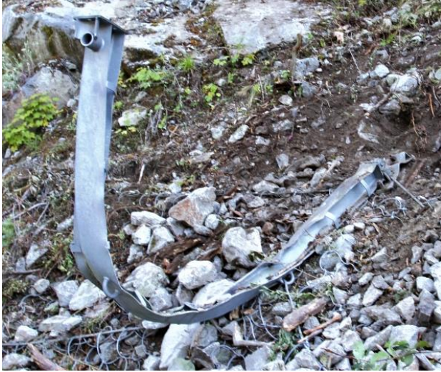
Figure 5. Post after removal of debris
