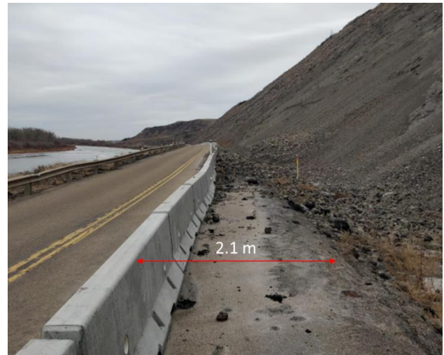
Figure 49. C018 rock slope Jersey barrier interim rockfall mitigation.
