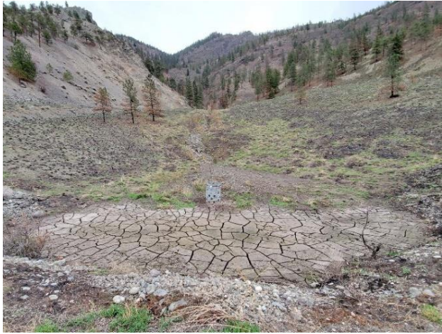
Figure 11. Sediment retention basin viewed looking upstream from the railway
