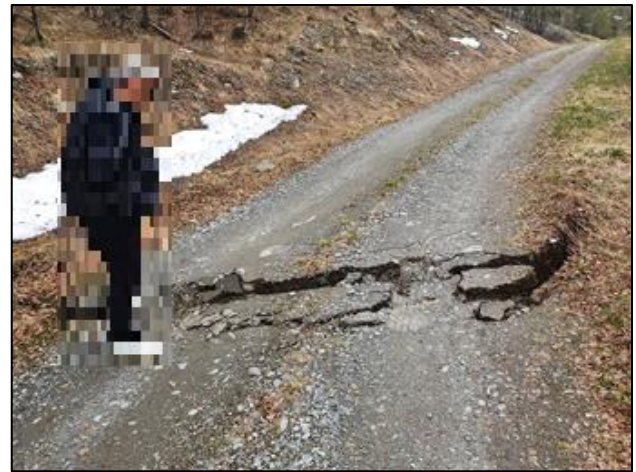
Figure 13. Large crack on access road to one of the houses one day before the landslide: location at failure surface upper edge on Fig. 11 (Photo courtesy Jan Egil Bakkeby)
