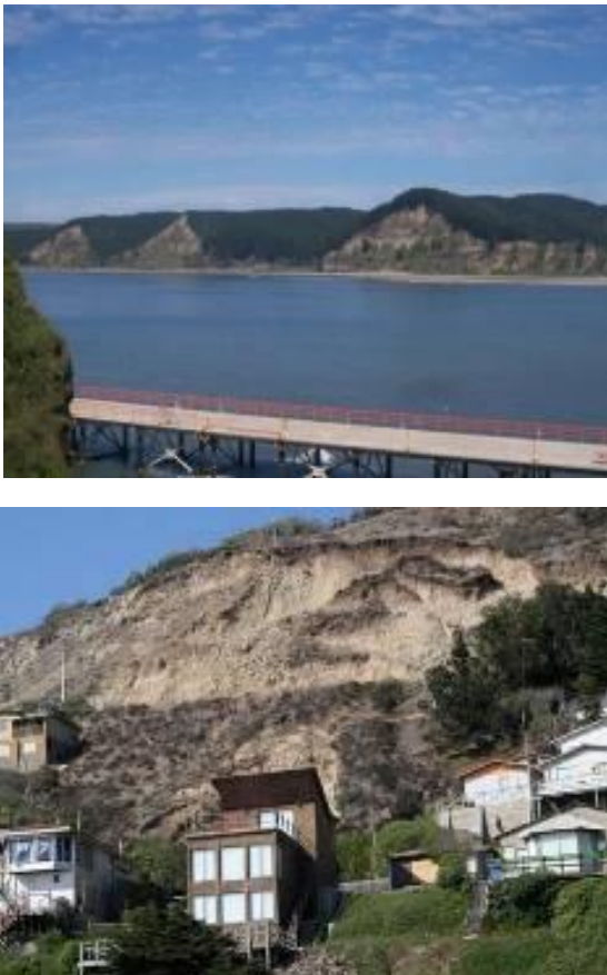
Figure 2. Coastal landslides triggered by the 2010 Maule earthquake in the Arauco peninsula (above, Moya 2016) and near Matanzas (below, Sepúlveda et al. 2012). Locations in Figure 1.
