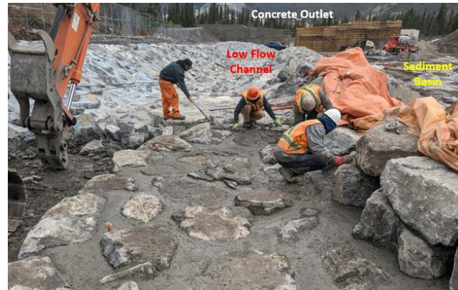
Figure 52 Grouted stone pitching in the low flow channel, looking downstream, during construction. The concrete outlet and berm are not yet built.
