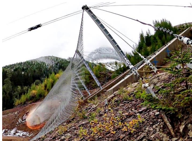
Figure 6. Maximum Energy Level test showing sparks during impact
