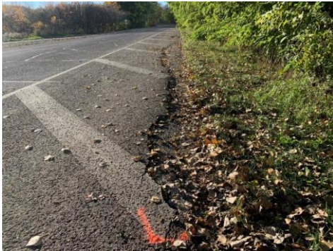
Figure 3: Photo of the tension cracks.
