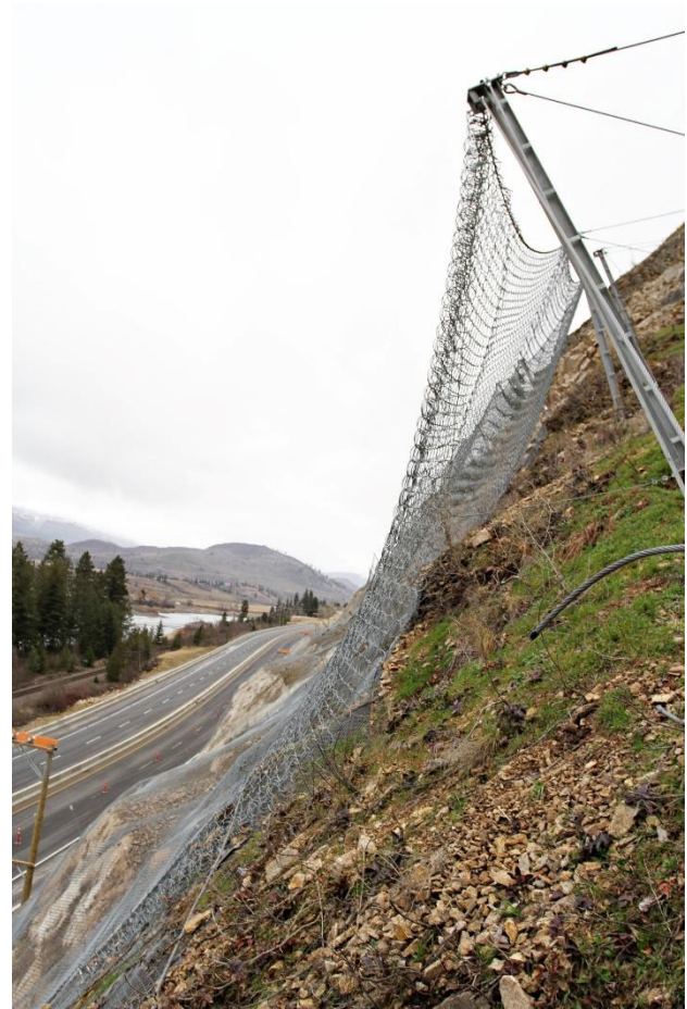
Figure 2. Attenuator system above highway.
