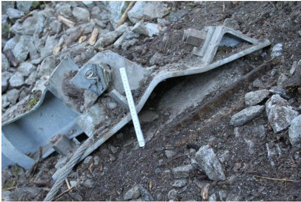
Figure 6. Deformed base plate
