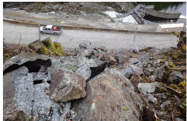
Figure 4. Slope impact point above fence
