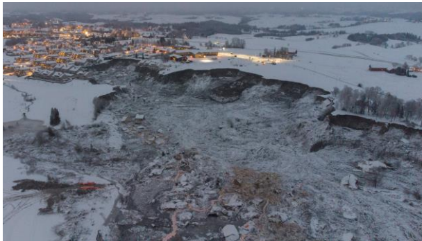
Figure 9. View of the Gjerdrum landslide (Norway) created by a retrogression in the sensitive clays (from https://www.uasnorway.no/europes-largest-drone-operation-after-deadly-landslide-in-norway-420-missions-and-200-hours-of-airtime/ ).
