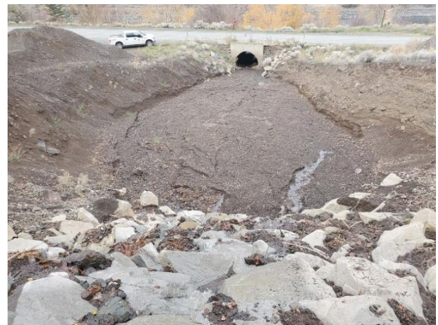
Figure 14. Sediment retention basin between the railway and highway
