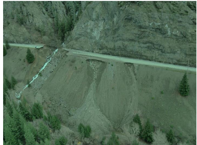
Figure 7. Washout of the Trans Canada Highway at Falls Creek. Photo by Tom Millard.
