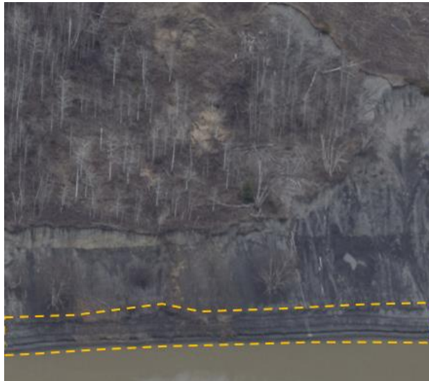
Figure 5. Shoreline on Site C headpond. Orange dashed line delineating evidence of wave-action after approximately seven months of headpond impoundment over an approximately 3 m elevation interval. Photo by M. van Veen, May 3, 2021.
