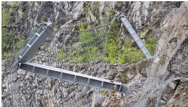
Figure 8. Bent post following direct impact
