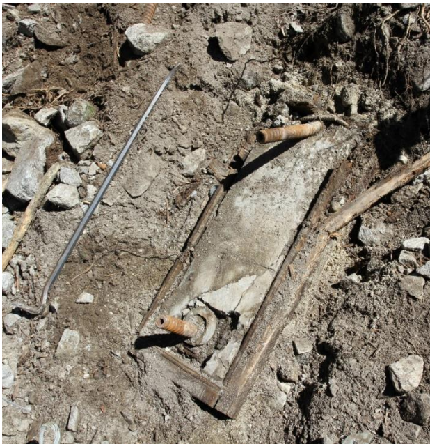
Figure 7. Post base support after 2011 impact
