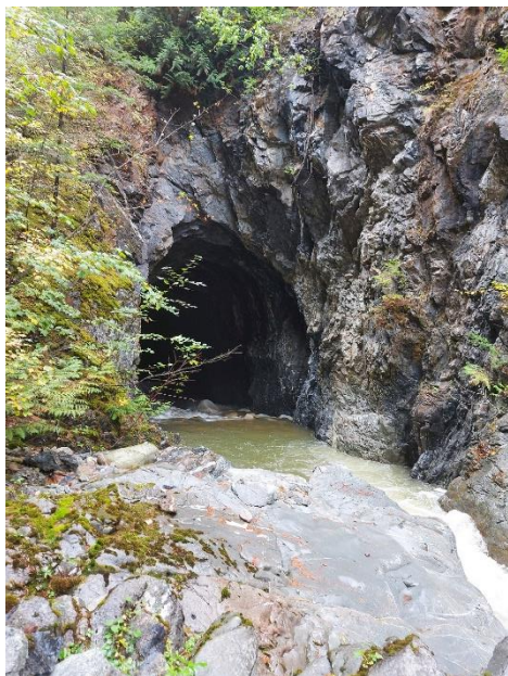
Figure 6. Entrance to the tunnel conveying Mowhokam Creek under Highway 1 and the CN railway. Photo by Tom Millard.
