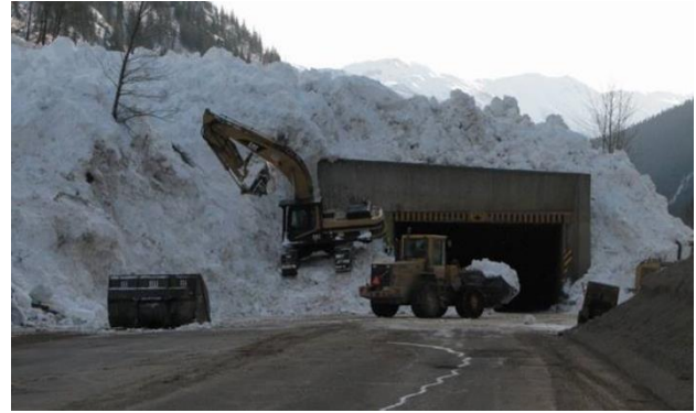
Figure 4. Mounds glide slab avalanche deposit, which buried the westbound portal of the Single Bench snow shed in April 2012 and resulted in a lengthy highway closure for deposit removal. Parks Canada photo.
