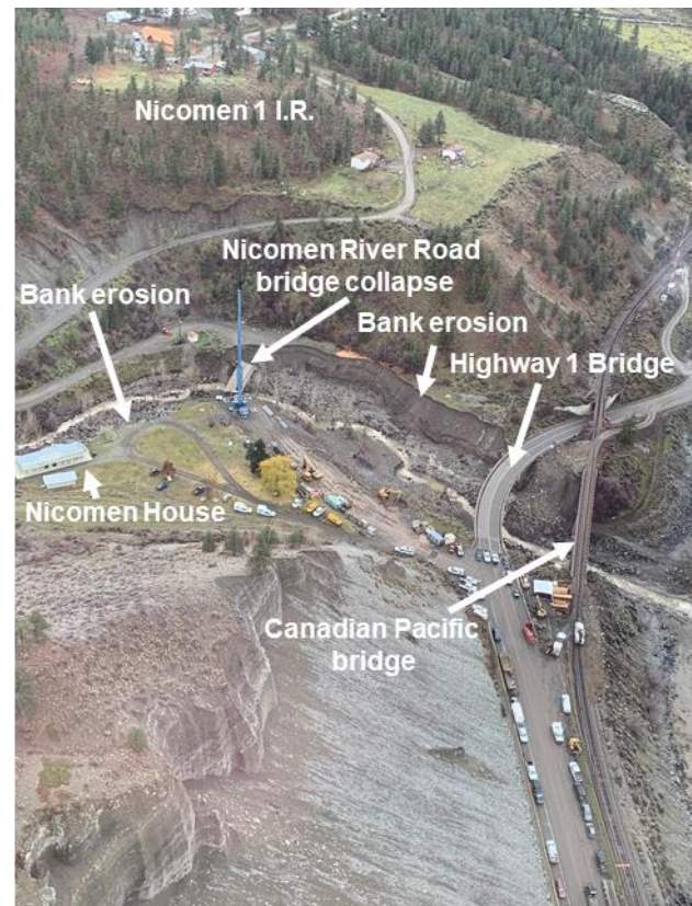
Figure 9. Looking south at the damage along Nicoamen River. The bank below the Nicomen House retreated by up to 10 metres from its pre-debris flood position. Photo by MOTI, annotations added by Carie-Ann Lau.
