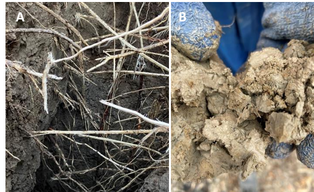
Figure 6 A) Roots within the embankment fill; B) Rootlets throughout the clay.
