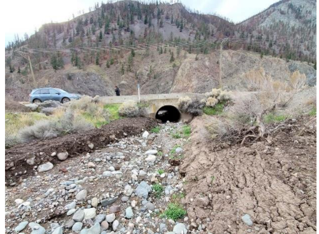
Figure 10 Drainage channel leading to Highway 1 and culvert under the highway
