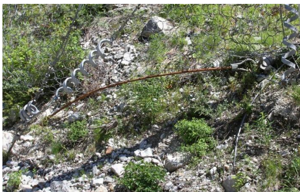
Figure 10. Pulled lateral anchor
